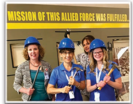
The Eisenhower Foundation staff grabbed hammers and hardhats to officially start the renovation project.
